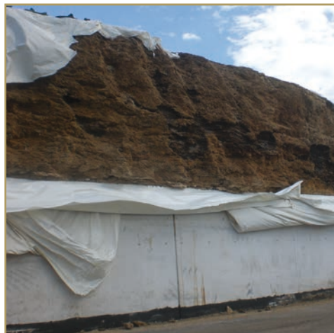
Picture 34: a) Overloaded silo in an Austrian biogas plant (left), b) oversized silo in USA (right, courtesy of Mr. Telmo Rodrigues)
