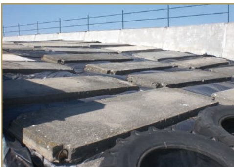
Picture 32: Silo covered with plastics sheets and a) bricks in El Salvador (top) and b) cement blocks in Czech Republic (bottom)
